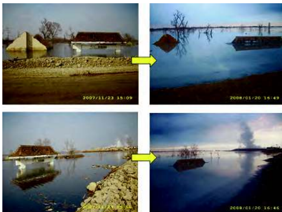
Fig. 27. Dramatical sinking of a village gate of Siring Timur, located to the west of the main vent. The gate and the rubble was half buried but still visible in the 23 November 2007 photograph. Two months later just a part of the tile roof and walls remain visible on 20 January 2008.
