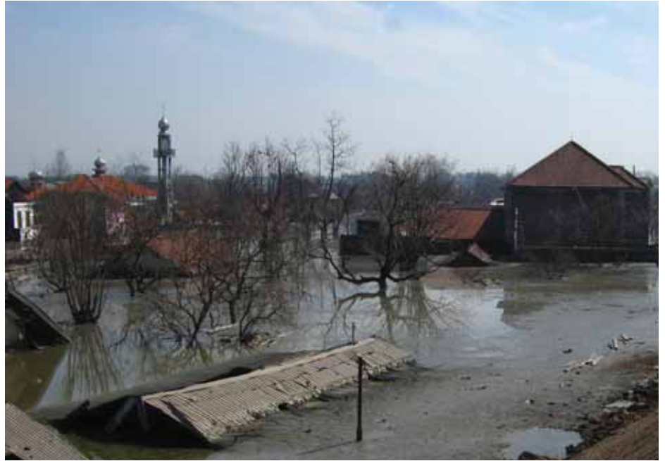
FIGURE 2. The impact of mud inundation. Note the depth of mud in relation to the building roof adjacent to the earth dam. Photograph taken 29th May 2007. © Atkins Ltd. 2007.
