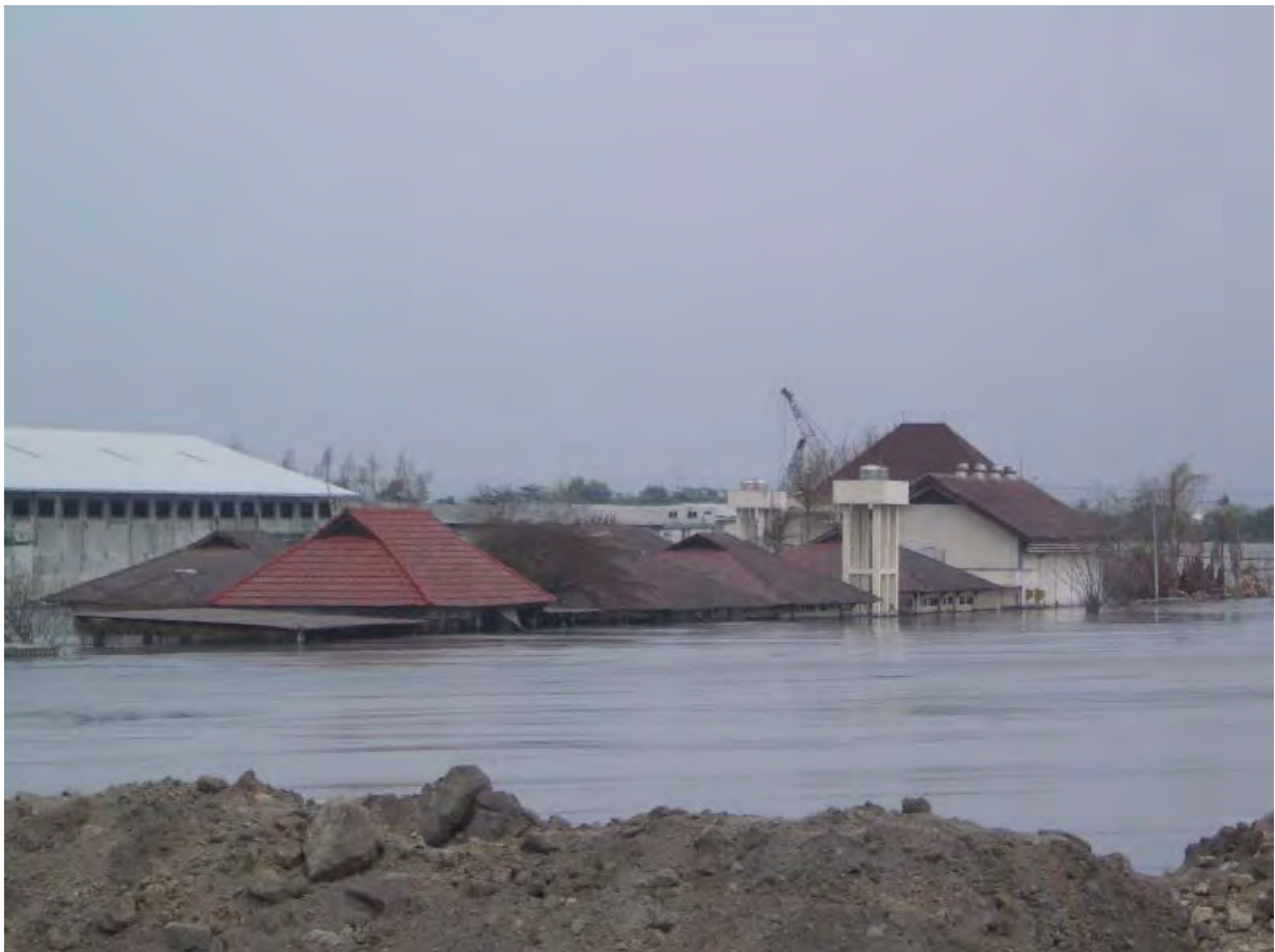
Buildings affected by the mud flows. Photo: R. Nijenhuis
